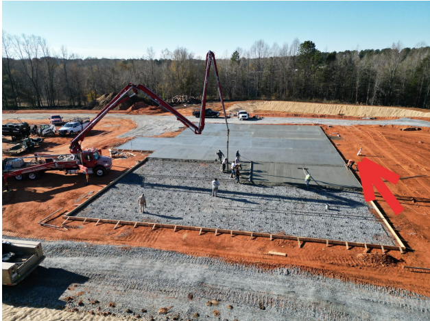
Photo shows measurements and markup added by the inspector.
